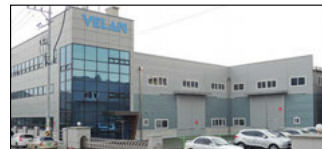
Ansan City, South Korea Velan Ltd., Plant 3
