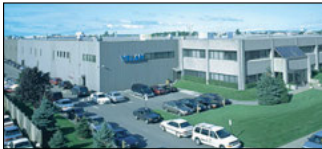
Montreal, Canada Velan Inc., Plant 2 and 7
