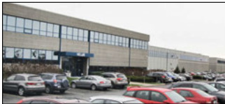
Montreal, Canada Velan Inc., Plant 5
