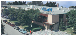
Montreal, Canada Velan Inc., Plant 1
