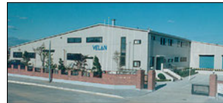
Ansan City, South Korea Velan Ltd., Plant 1
