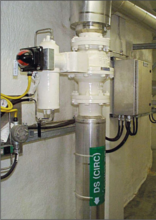
Split-body ball valves installed in a waste water treatment plant in Canada.
