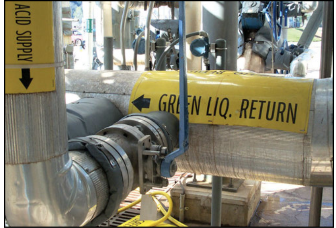
Split-body ball valve in pulp and paper.
