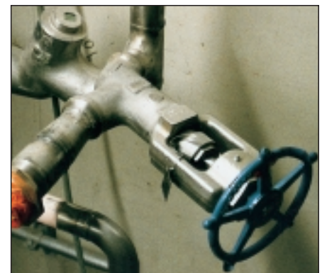
Class 2500 hermetically-sealed Y-pattern bellows sealed valves.
