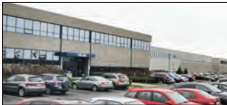
Montreal, Canada Velan Inc., Plant 1 and 5
