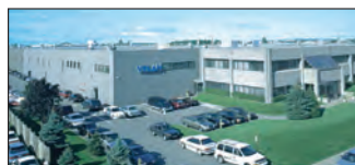
Montreal, Canada Velan Inc., Plant 2 and 7
