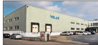
Ansan City, South Korea Velan Ltd., Plant 2
