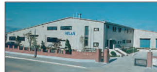
Ansan City, South Korea Velan Ltd., Plant 1
