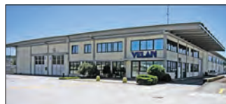
Lucca, Italy Velan ABV S.p.A., Plant 2
