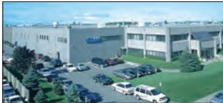
Montreal, Canada Velan Inc., Plant 2 and 7
