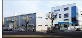
Ansan City, South Korea Velan Ltd., Plant 1
