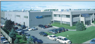
Montreal, Canada Velan Inc., Plant 2 and 7
