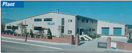
Ansan City, South Korea - Velan Ltd. Plant 1 - 20,000 sq. ft. (1,900 m 2 ) Cast steel gate, globe, and check valves
