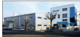
Ansan City, South Korea Velan Ltd., Plant 1
