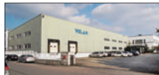
Ansan City, South Korea Velan Ltd., Plant 2
