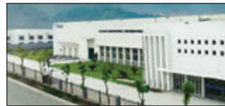
Suzhou, China Velan Valve (Suzhou) Co., Ltd.
