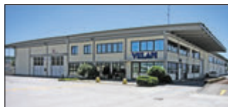
Lucca, Italy Velan ABV S.r.l., Plant 2
