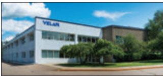
Williston, VT, U.S.A. Velan Valve Corp., Plant 3
